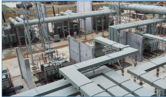
SEGREGATED/NON-SEGREGATED PHASE BUSDUCTS (415-33 KV UP TO 6500 A)
